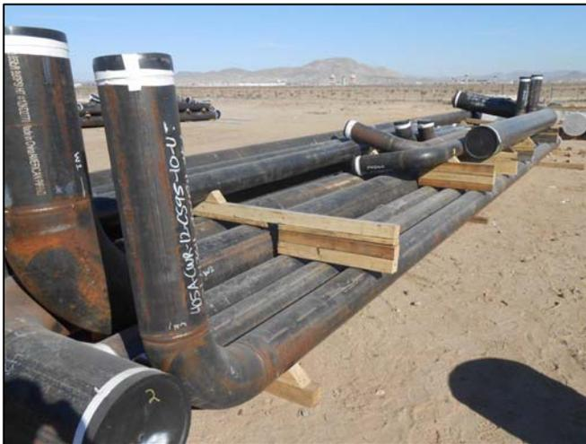
**Figure 3: Pre-fabricated pieces save time and money** allowing the installation process to require fewer welds and less painting in environments where quality is not easily controlled.
