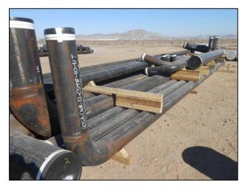
Figure 3: Pre-fabricated pieces save time and money allowing the installation process to require fewer welds and less painting in environments where quality is not easily controlled.
