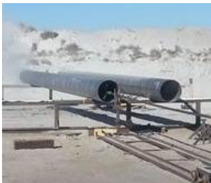
Internal blasting SP10 Near White Metal. Blast Profile: 1.5-3.0
