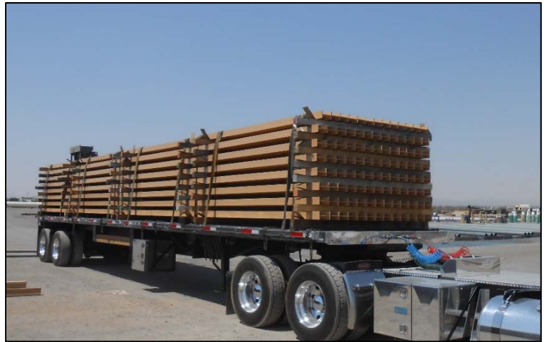
H-piles for a solar facility near Calipatria, CA - the coating was applied as 20 mils nominal thickness with pile length varying from between 13-25 feet depending on the structural load requirement
