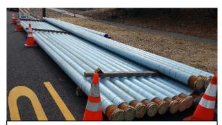
The annual pipe contract includes cement mortar lining for drinking water applications. In addition to supplying a custom blue color for EBMUD, Seal for Life, manufacturer of Synergy™ also provided a two year warranty for UV protection. It provided an additional six months versus the other coating option.
