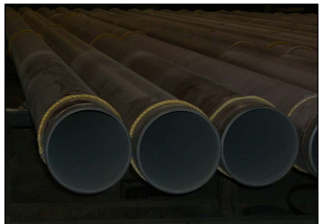
12-inch pipe blasted and ready for the Enviroline® 405HT-LV lining. Pipe was blasted per SSPC SP-5/NACE #1 white metal standard.
