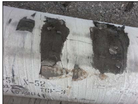
The Existing Coating Prior to Mobile Pipe Repairs
